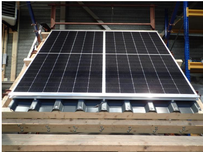
Photo 8 The PV modules have been positioned in the insert profiles.
