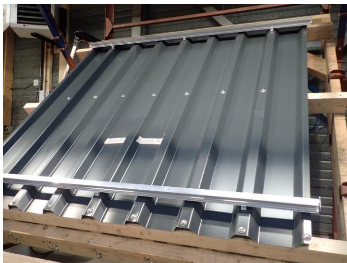
Photo 5 Two insert profiles have been fixed to the IP-Fix clips.
